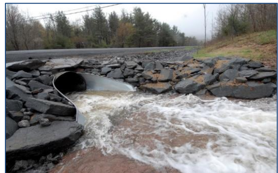
Enlarged culvert and added inlet walls to focus water flow away from roadway.
